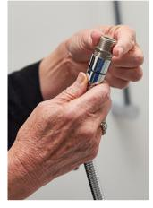
**3)** Take the stainless steel barrel and screw it into the tapered end of the hose.
