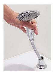
**1)** Start by pulling out the hand shower from the deck of the tub.
